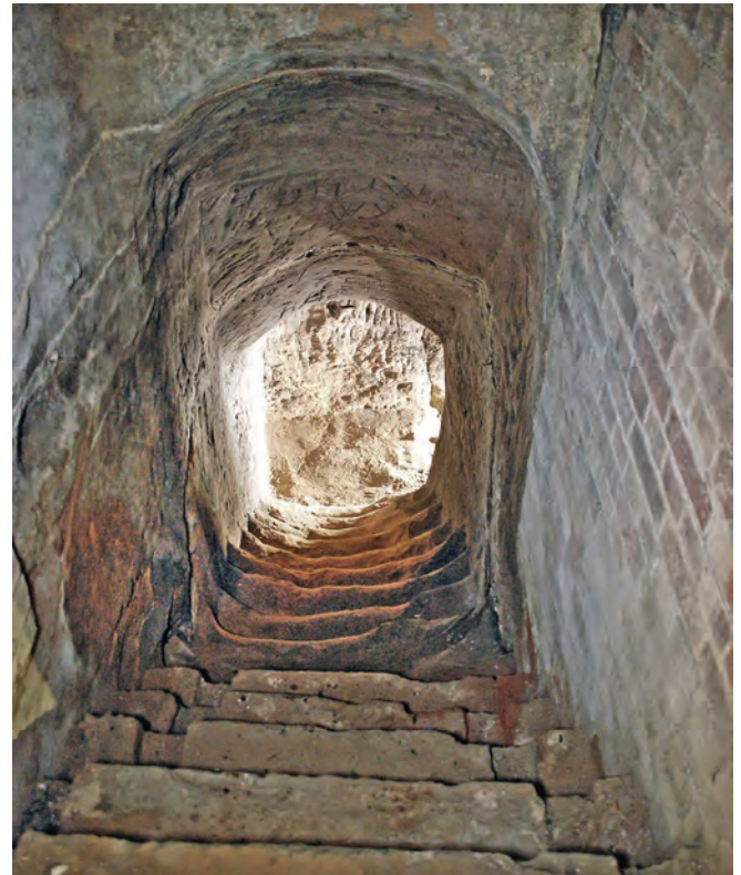
Stairs down from the cellar to the well passage
